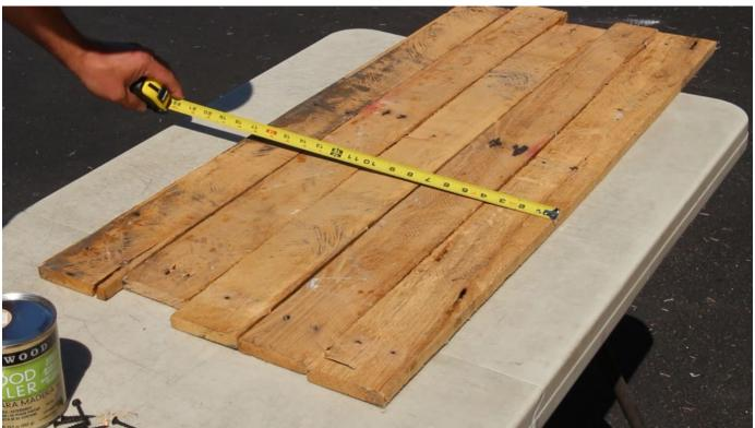
**Step 3:** Using a <u>tape measure</u>, measure and mark your wood pieces to lengths of about 24" each. Cut the wood on the marks using a <u>circular saw</u>. Using a <u>wood clamp</u> will come in very handy when cutting the wood. Simply clamp the material down to your table to help safely keep the wood in place.
